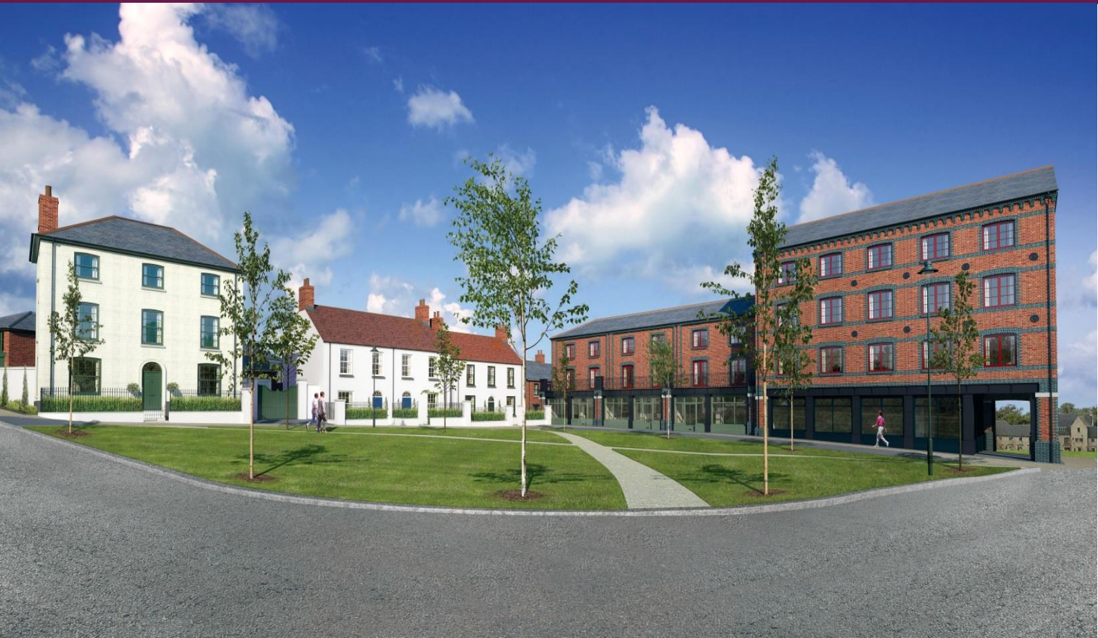
CGI impression. Units under construction.
