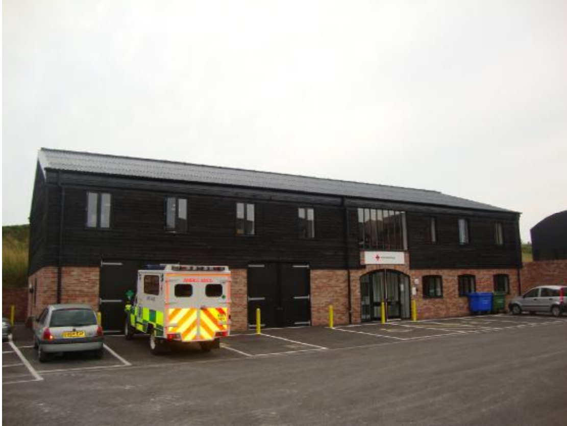
PHOTO SHOWS UNITS 5A AND 5B (WHICH ARE NOW LET)
